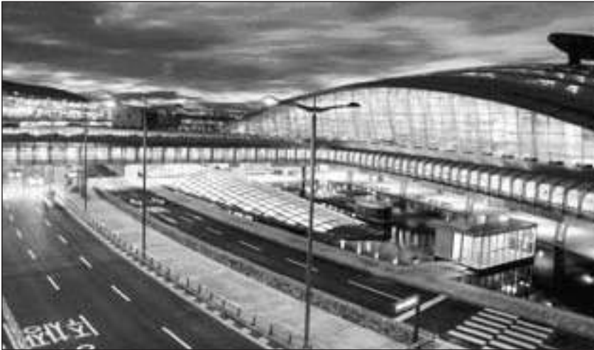
Incheon International Airport
